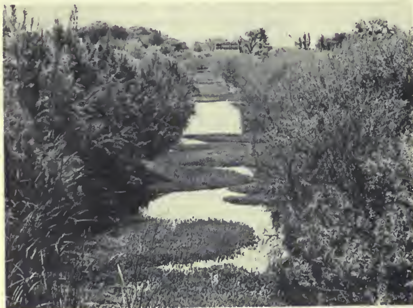
PARROT FEATHER covers drain from side to side in many places on Rio Grande project. Cattails, Salt Cedar, and willows can also be seen in this photo, taken by Fred S. Finch, Region 5.
